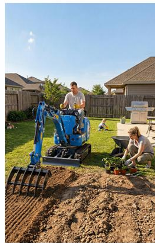
LEVELING THE LAND
